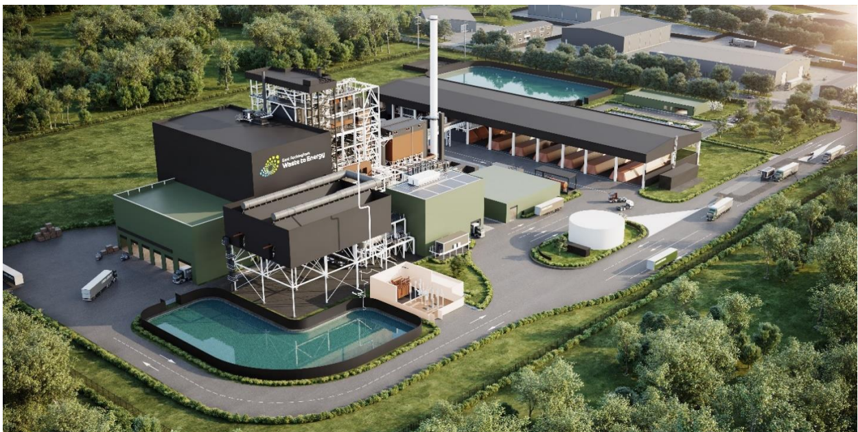
The East Rockingham facility will be Australia's first large scale thermal energy-from-waste operation, with capacity to process 300 kt of waste per year and generate 29 MW of energy. Image kindly provided by East Rockingham Waste to Energy
