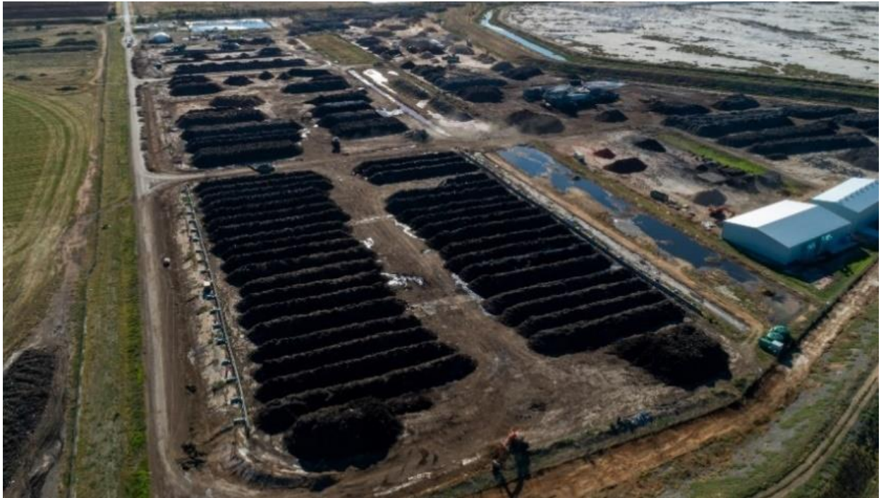
Photo 7 Aerial view of compost windrows at Jeffries in South Australia
